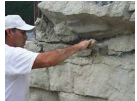
Expertise is required to blend and color the castings into a continuous formation.
