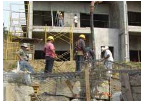
Concrete backfill ensures a permanent structure that will last many decades.
