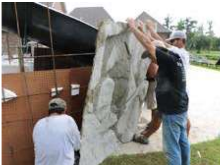
RicoRock panels or boulders are secured to a rebar armature for most applications.
